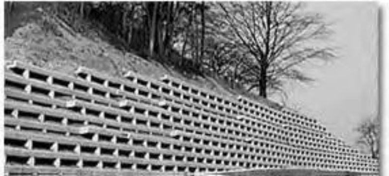
Parkway Retaining Wall - Post Construction
